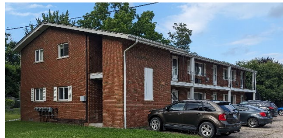
Six- Unit Housing near Downtown Area
